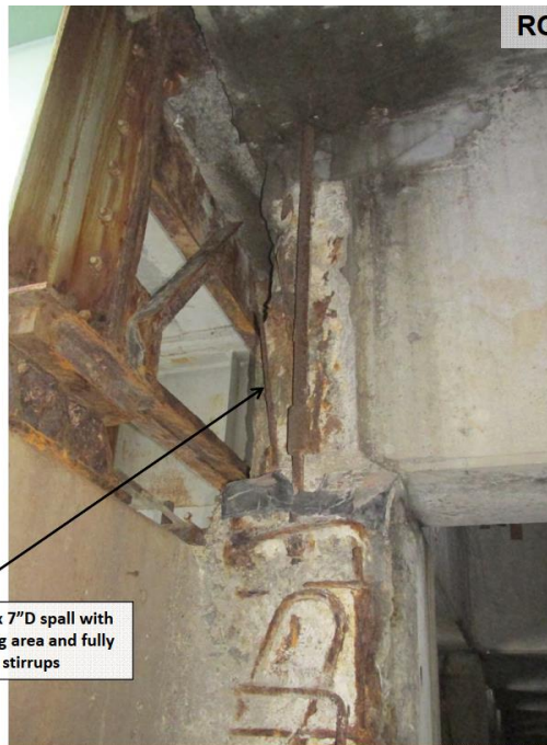
Figure 27. Inspection photo of exterior tie-down rod for cantilever beam A at Pier 6 taken July 2015 (AECOM).
