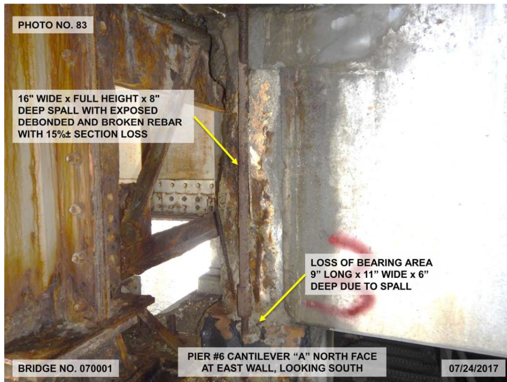
Figure 29. Inspection photo of exterior tie-down rod for cantilever beam A at Pier 6 taken July 2017 (Collins).
