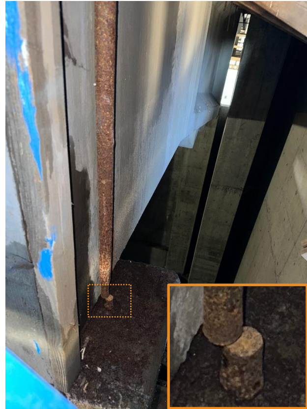
Figure 2. Pier 7 Cantilever F fractured tie-down rod
