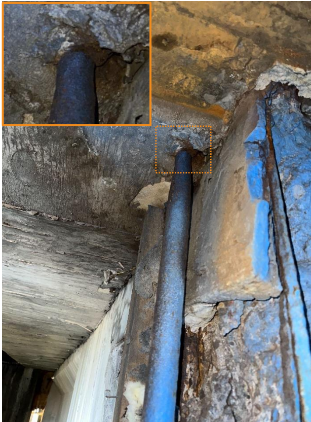
Figure 1. Pier 7 Cantilever A fractured tie-down rod
